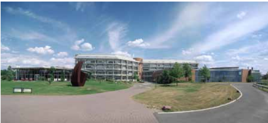
BfR - Federal Institute for Risk Assessment, Berlin-Marienfelde, GERMANY
